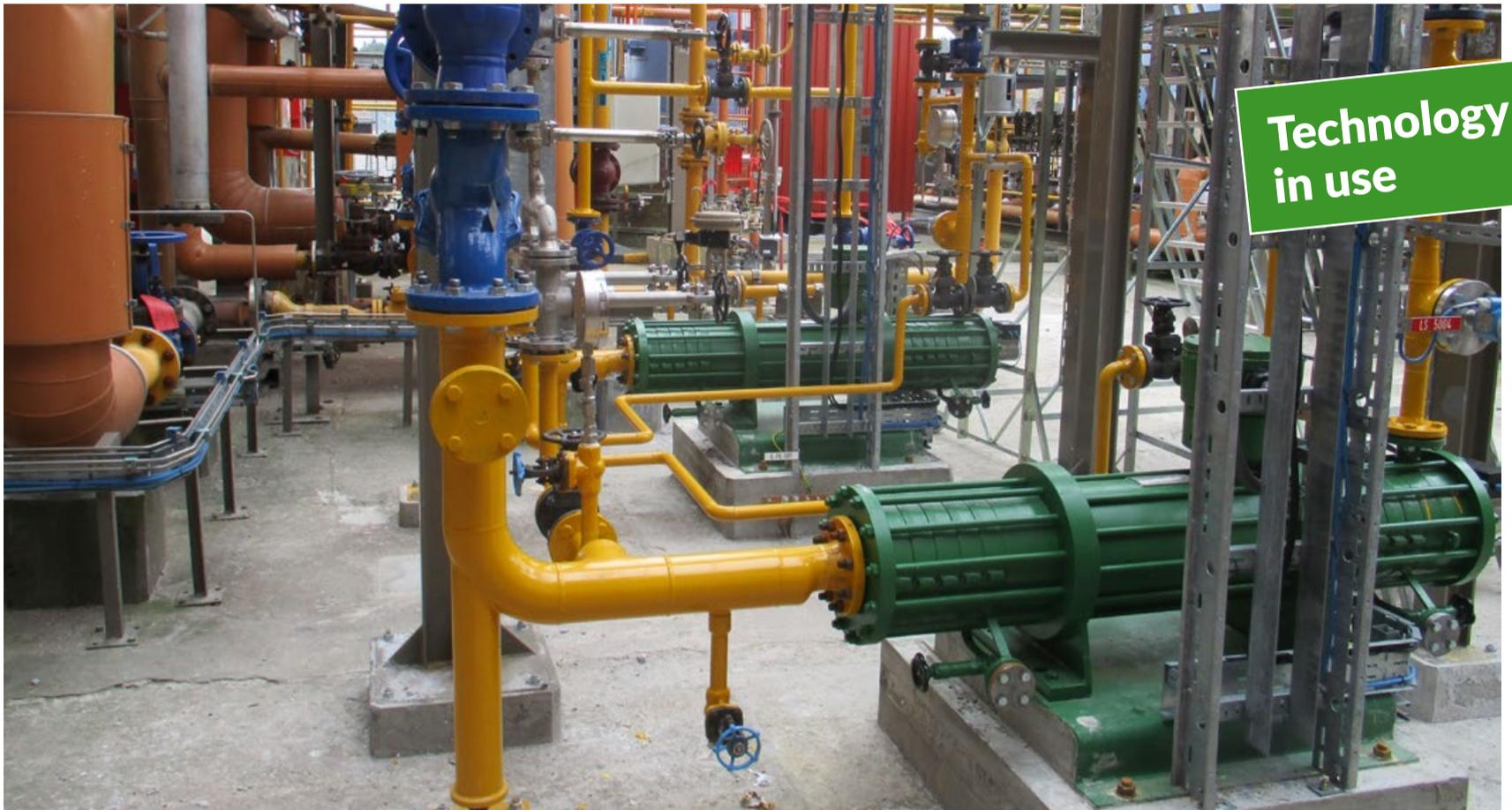
Canned motor pumps with tandem design
