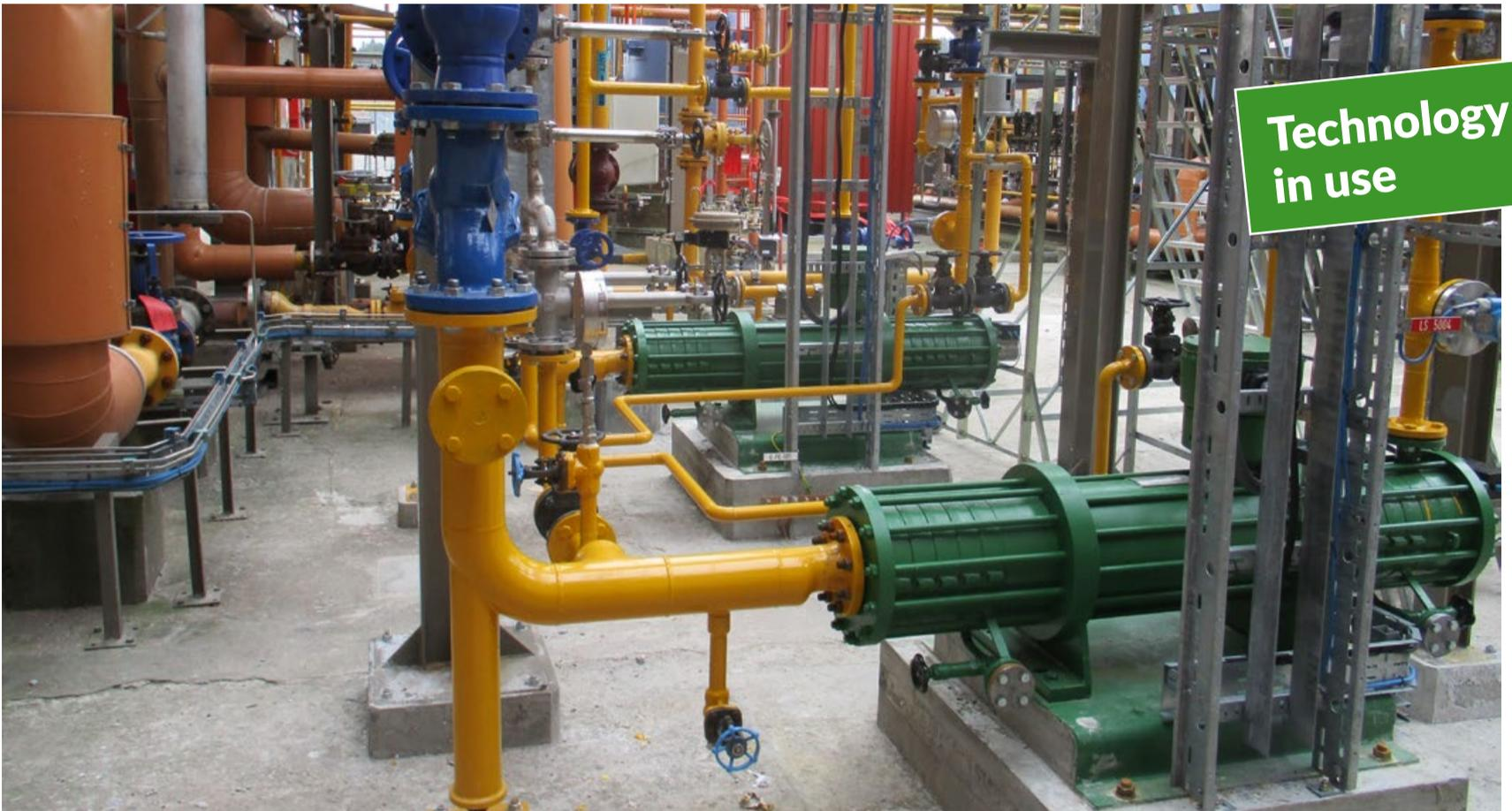
Canned motor pumps with tandem design
