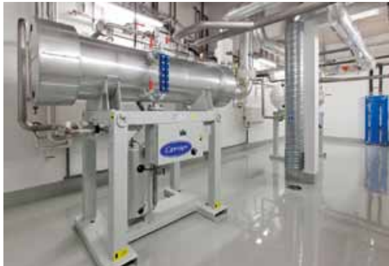
Heat exchanger (CARRIER)
