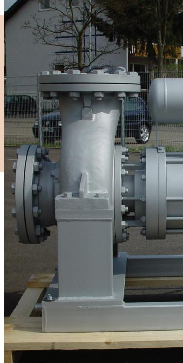
API 685 is the new standard for sealless centrifugal pumps.
