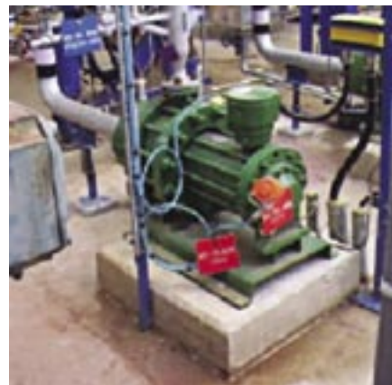
FIG. 3 Typical canned motor pump installation.
